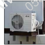
AC COMPRESSOR INSTALLATION ON EXTENDED SKID OF THE CABIN
