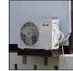
AC COMPRESSOR INSTALLATION ON EXTENDED SKID OF THE CABIN
